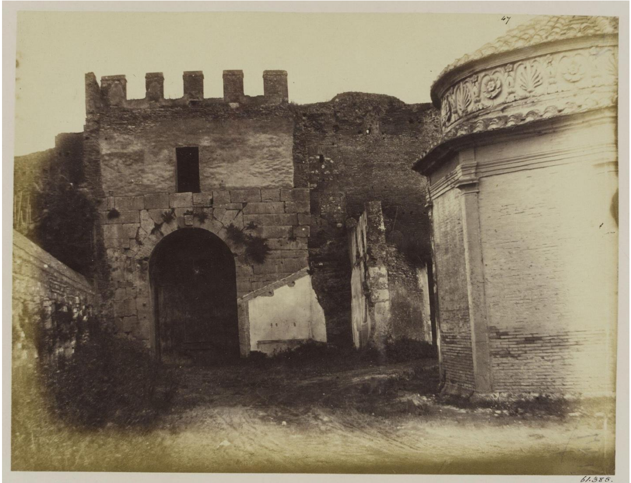
Parker, John Henry. No 67. (V&A). "Porta Latina closed and Chapel of St. John Olio". The stone, brick work and crenelated cap have been captured per instructions in this image but so too the Chapel and the carriage tracks contextualizing the gate into its urban space.
