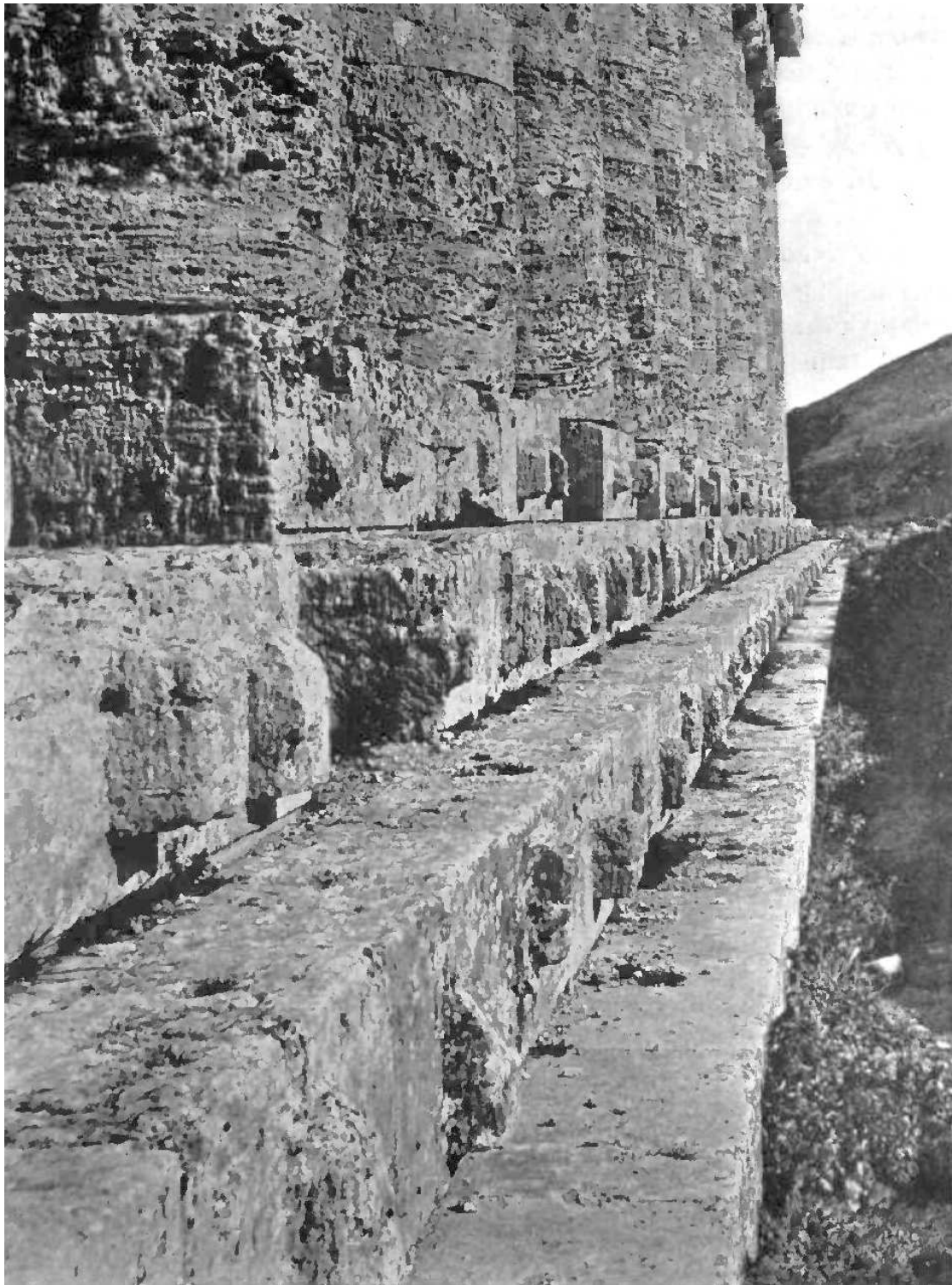
n°18 – Flank of Temple at Segesta – showing curve of Stylobate and bosses for lifting the stone
