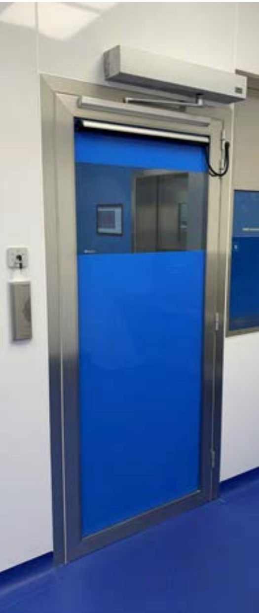
Automatic hinged door section with decus connection
