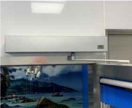
Automatic swingdoors engine
