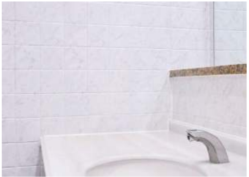
Restroom refurbishment / ST-024TIL
