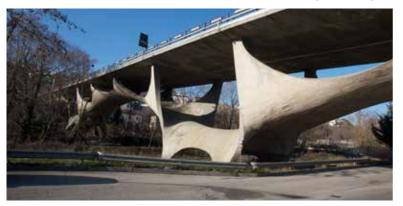
bridge in Potenza, the *Musmeci*. Designed in the late 60's by Eng. Sergio Musmeci, stands out in the Italian engineering scenario for the particular combination of functionality and plasticity of the structure. Its design is quite singular: a single vault with a thickness of only 30 cm is supported by 4 spans whose profile recalls that of a huge, crumpled leaf, whose tips act as support pillars.
