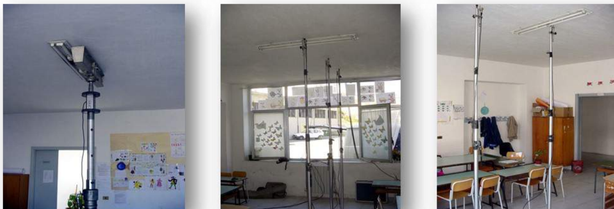
Loading tests on the floor
