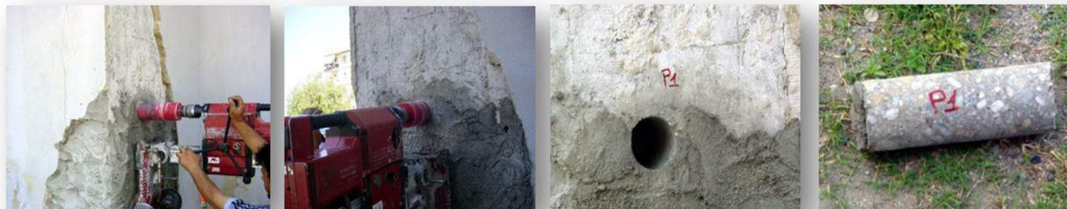
Extraction of concrete cores
