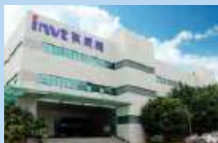
Shenzhen Fuyong Industrial Park
