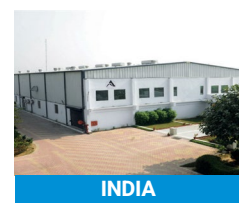
Autotech Sirmax North - Palwal PP Compound
