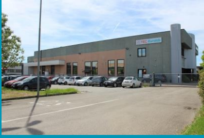
TEC Eurolab Srl - Headquarter (Material Testing Centre): Viale Europa 40 41011 Campogalliano (MO) - ITALY
