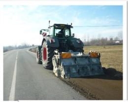
SERREMAR ITALIA has self-loading cutters, capable of milling the surface layer of the road surface for about 02 - 30cm and preparing the surface for the new asphalting.
