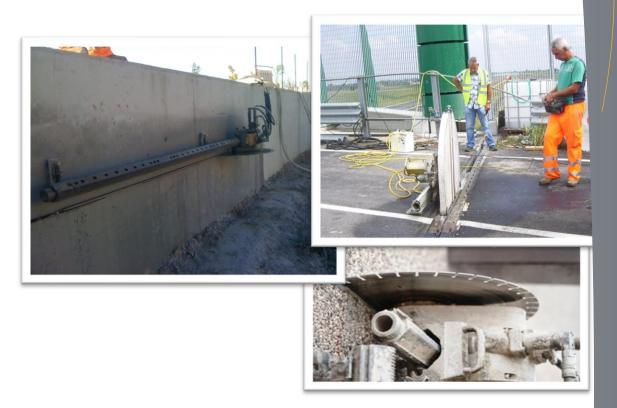
The technique of **cutting walls** and **cutting of reinforced concrete** is widely used in all cases of partial, civil, industrial and controlled demolition of masonry and, above all, in restructuring and restoration situations where precision and containment of vibrations with low emissions are required. of pollutants, such as noise and dust.
