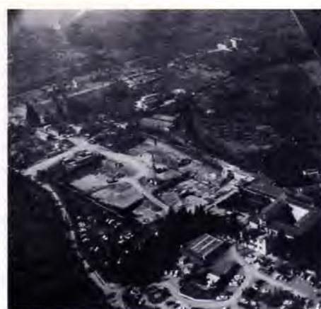
Foto aerea a scavo ultimato / Aerial view of the completed digging
