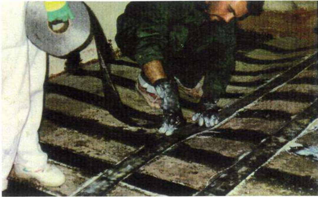
(Some application phases of the carbon reinforcement)
