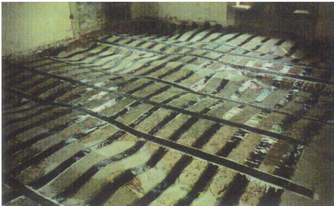
(Vault surface after reinforcement with carbon fibers sheet applied with epoxy pade)
