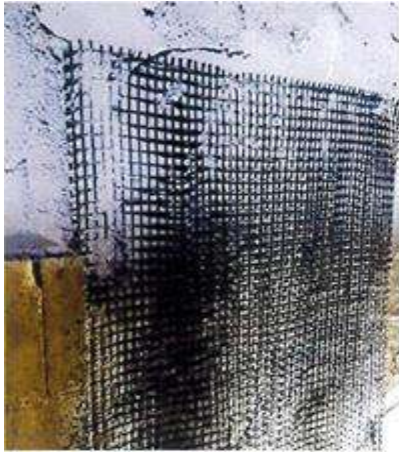
NATURAL HIDRAULIC LIME PLASTER REINFORCED WITH CARBON FIBER NET
