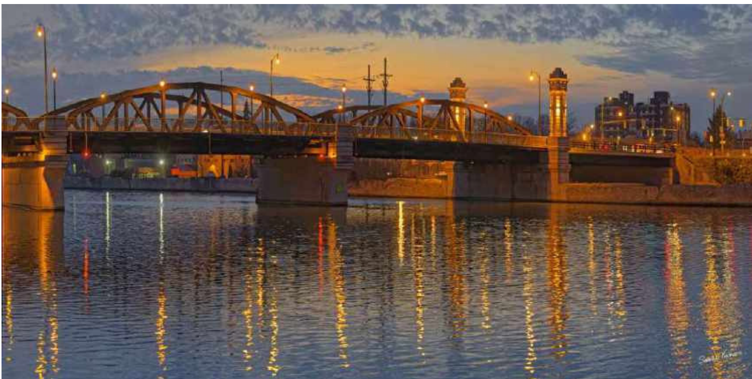
Ford Street Bridge (2020)
